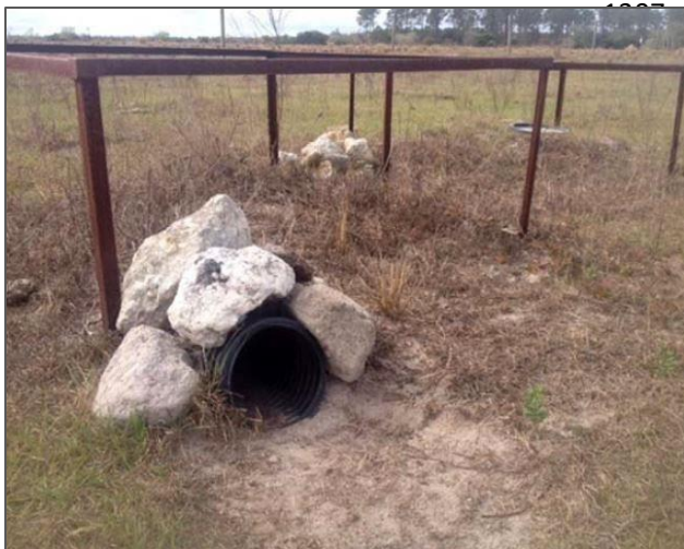
Figure D-1. Metal device used to prevent collapse of artificial burrows while allowing full access for cattle to graze. Photograph by Quest Ecology, Inc.
